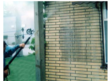
CLEANING YELLOW CEMENT BRICKS
